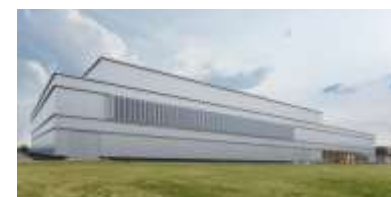
Neubau Physical Fitness Center, Katterbach
