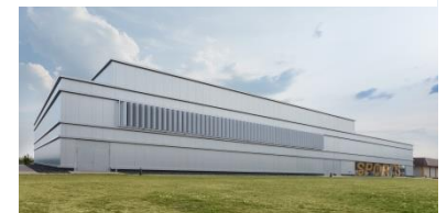
Neubau Physical Fitness Center, Katterbach
